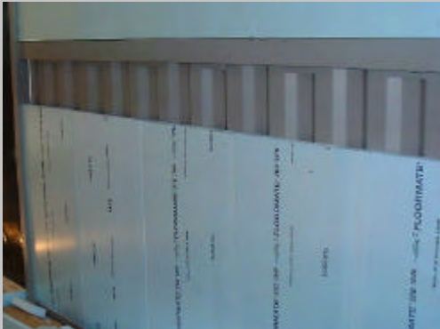
Stage 3 Container thermal insulation and lining
