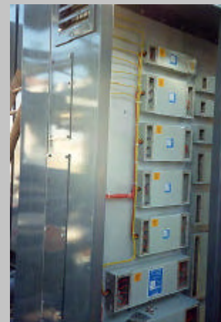
Stage 5 Installation of Tempest filters
