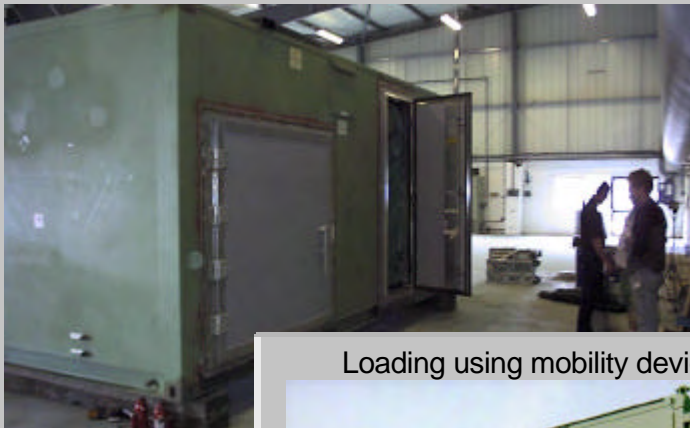
Stage 4 Fitting RF shielded doors
