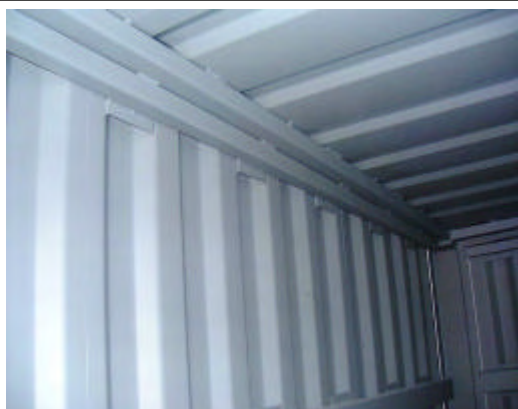
Stage 3 Container interior coated with anti corrosion paint
