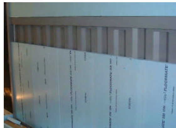
Stage 4 Container thermal insulation and lining
