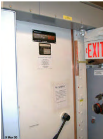
Stage 7 Completion of internal equipment
