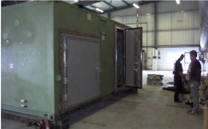
Stage 5 Fitting RF shielded doors
