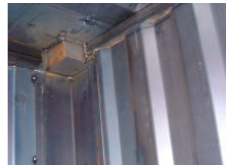
Stage 2 Construction All joints fully welded
