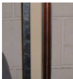
Double row of copper beryllium finger contacts on door frame
