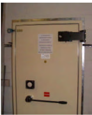
RF shielded double knife edge door with 4 point latching and double action hinges.
