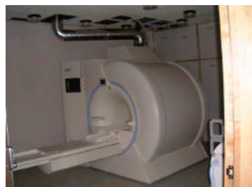
MRI suite after installation of internal linings and the scanner
