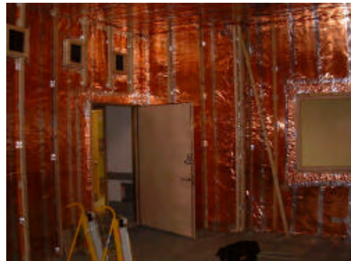
MRI suite during installation
