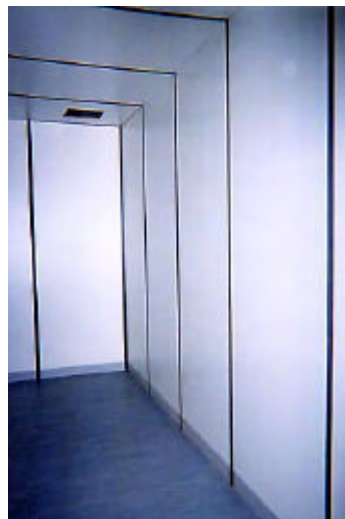
Modular room under construction
