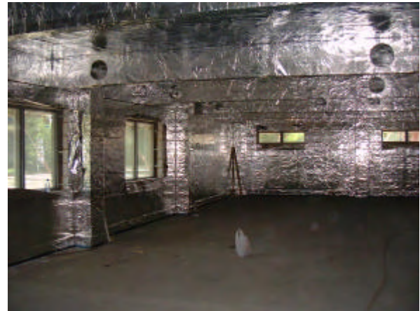
Internal view of room during installation of foil
