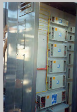
Stage 5 Installation of Tempest filters
