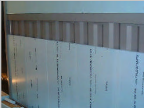
Stage 3 Container thermal insulation and lining
