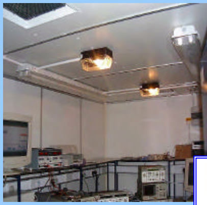
Internal view of chamber showing lining and fittings
