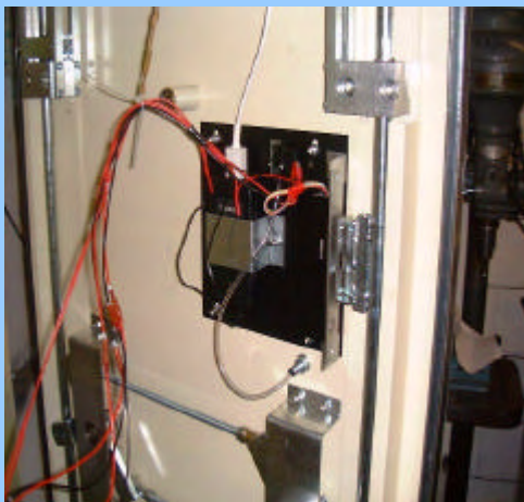
Internal view of door showing 4 point latching mechanism and electrically operated solenoid lock
