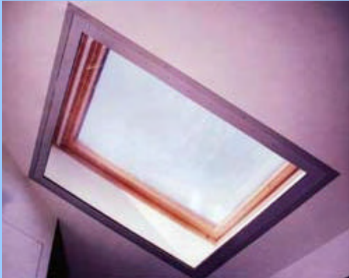
Example of secondary RF shielded window in laboratory
