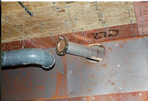
Pre-positioned pipe end to match MRI cryostat pipe
