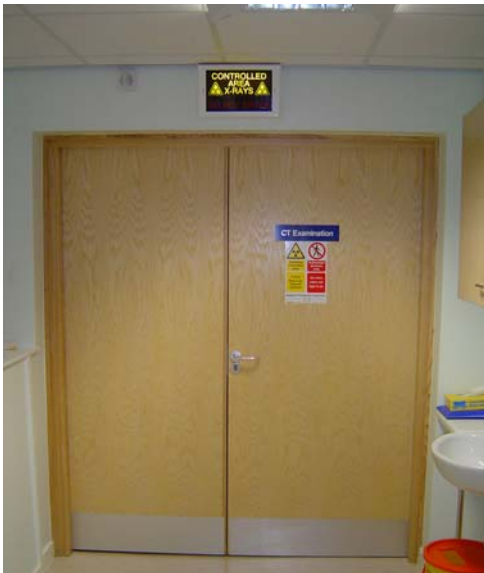
Ash veneered lead lined door for CT scanner room
