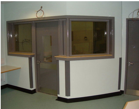
External view of veterinary X-Ray room showing leaded windows and door
