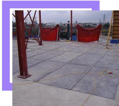
EMF Steel screening installed on the floor to prevent interference from electrical substation below the floor
