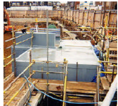
Complete sub station enclosed in EMF steel screening, to prevent low frequency fields affecting living accommodation in housing to be built above.
