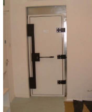
RF shielded single knife edge door with 2 point latching on modular steel room
