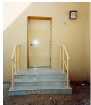
RF shielded door modified for external use
