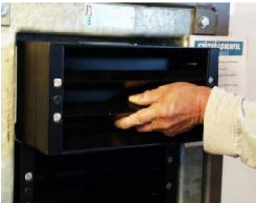
Mounting blast valve module (Item B) into frame (Item A)
