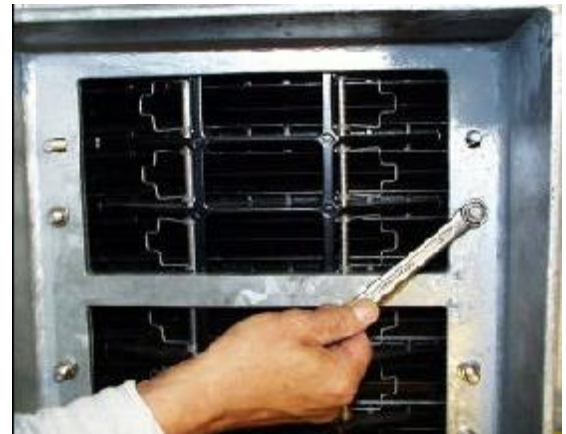
Tightening blast valve unit (Item B) into the frame (Item A)
