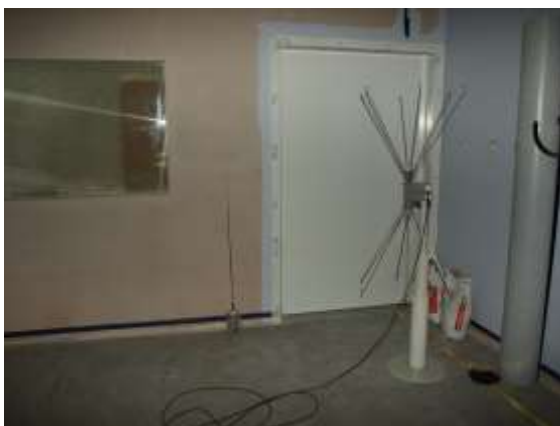
RF shielding attenuation test on MRI chamber
