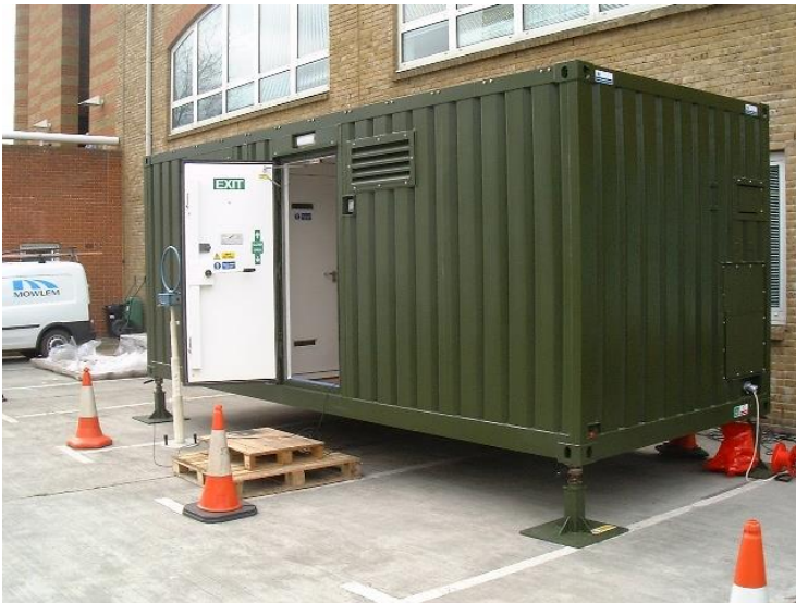
Shielded Door Fitted to Container
