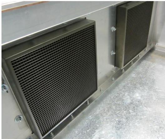
Steel square matrix 10 mm x 50mm used to form WGBC for air ventilation
